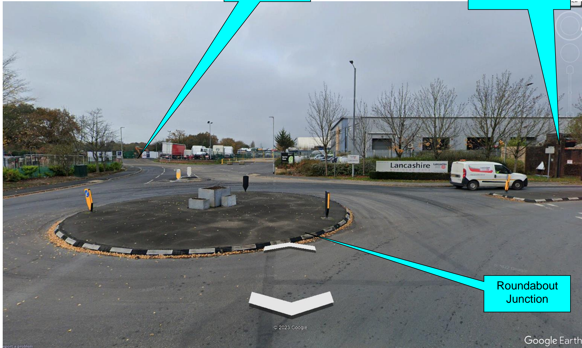
View looking towards Site Access Road
